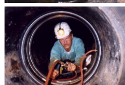
Pressure Test Seal
