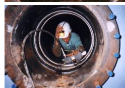
Expand Bands with Expander
