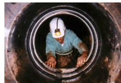
Install Retaining Bands
