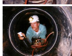
Check for Leaks
